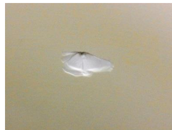
Damaged gun ceramic
