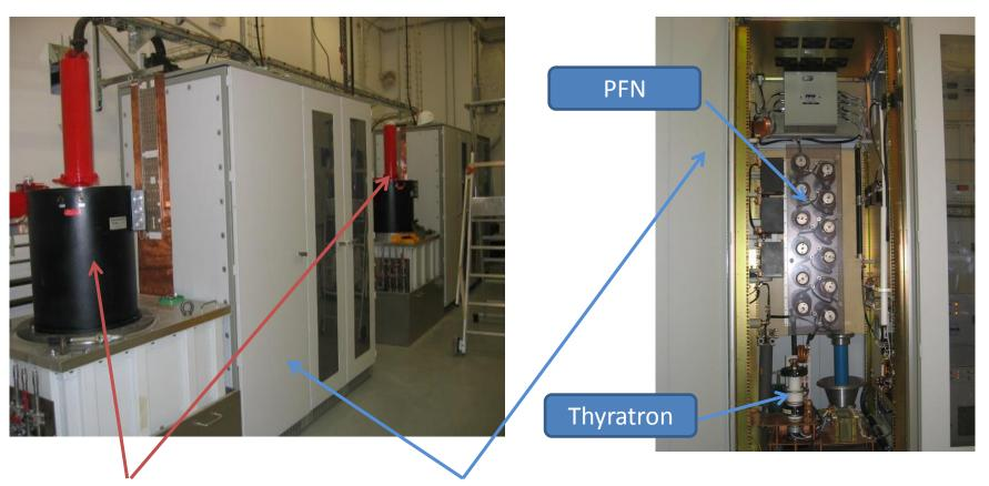
2 x 35MW TH2100 Klystrons & HV modulators (300kV, 280A, 6μs pulse at 3Hz) 1<sup>st</sup> klystron feeds buncher + accelerating section1 & 2<sup>nd</sup> klystron accelerating section2
