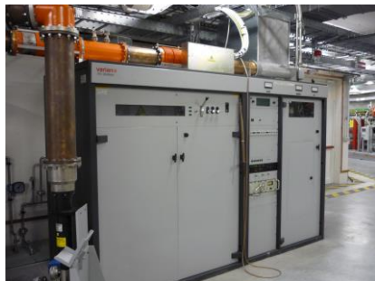
60 kW klystron-based Tx
