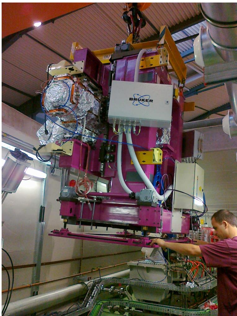
**Figure 1. IDs:** A snapshot taken during the installation of the in-vacuum undulator 1 (IVU-1).
